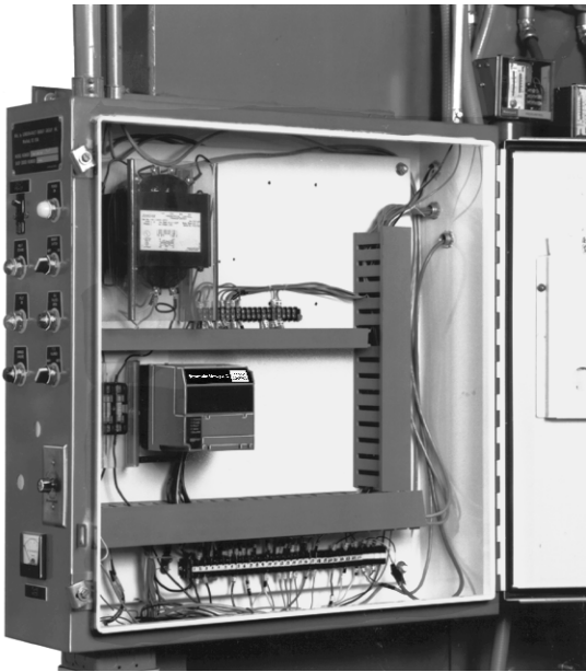
Fig. 7. Electrical panel installation.
